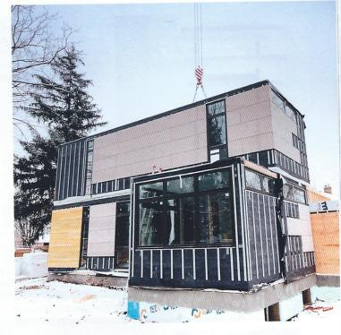
↑ The house is fully kitted out with green features, including geothermal heating and cooling. The exterior uses a fibre cement rain screen system that helps prevent leaky house syndrome.
